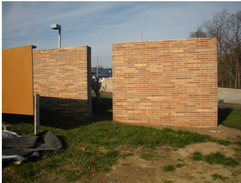
Figure 9: Mock-up of Original Face Brick
