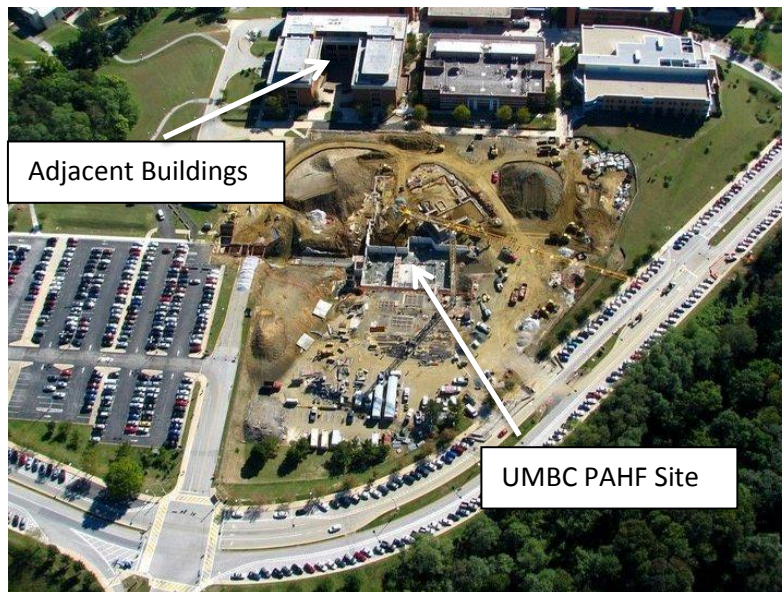
Figure 7: Aerial View of UMBC PAHF Construction Site
